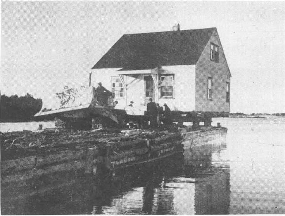
TWO-STORY "PRE-FABS," built during the World War, are being moved from Pictou to provide comfortable, sanitary quarters for Indians on reservation. Old, run-down dwellings in Indian community will be destroyed.
